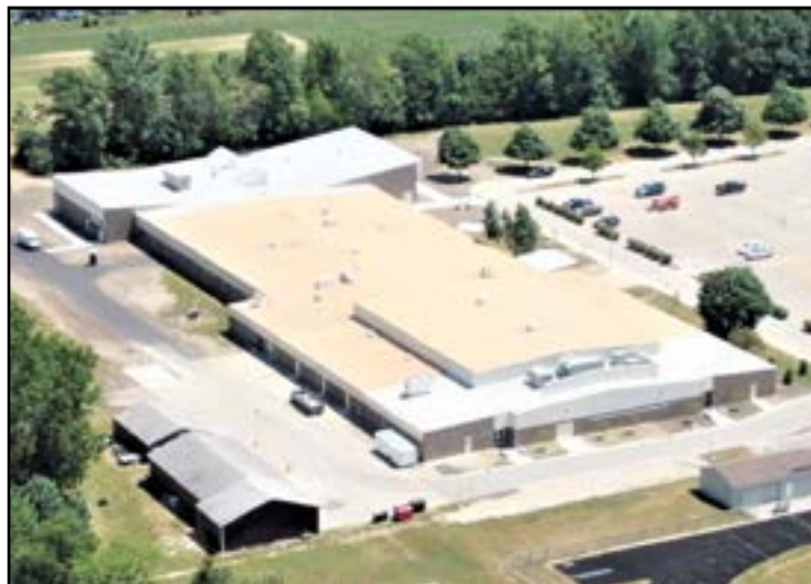
This aerial photo (looking east) provides an excellent view of our recent additions to the west end beyond the existing gymnasium and the new classrooms on the east end of the building (drone photo taken June 2020).
